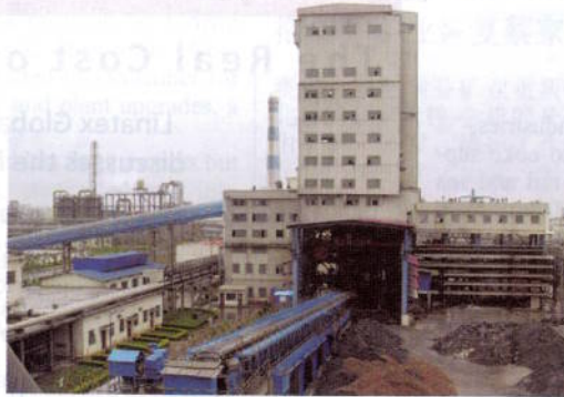
The Qujing ISA-YMG plant with casting machine.
