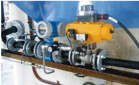
Left – The recently released IsaCharger™ being used to charge IsaMills™ automatically to maintain power set point with no moving parts
